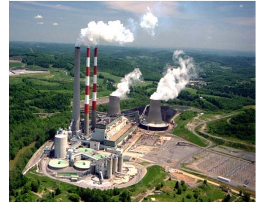
1984MW, Supercritical Harrison Power Station, West Virginia, USA.
