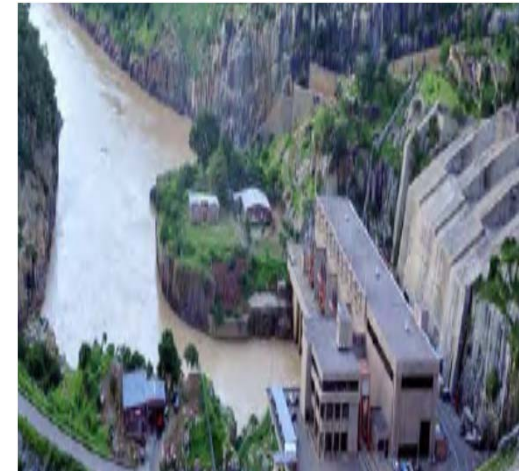
Shiroro Hydro Electric Power Plant, Nigeria
