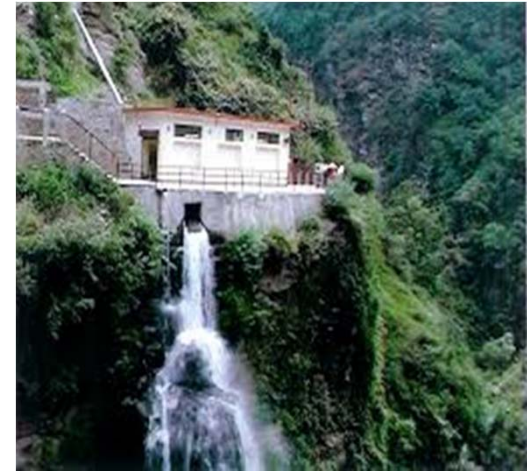
Small Hydro Power Plant
